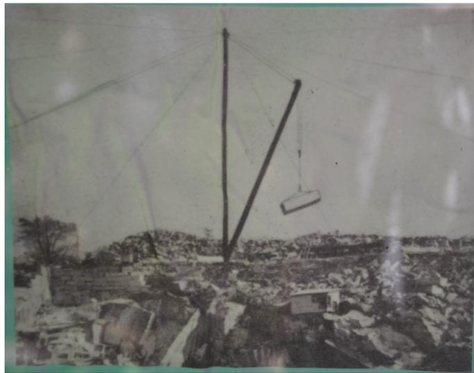
The remains of the derrick (left) used to lift the cut granite and what it looked like in operation (above) with the boom (no longer present) attached.
